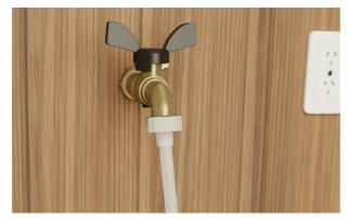
**3.** Ensure the rubber washer is fitted when connecting the inlet hose to the tap. Hand-tighten into place.
