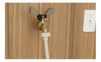
**3.** Ensure the rubber washer is fitted when connecting the inlet hose to the tap. Hand-tighten into place.
