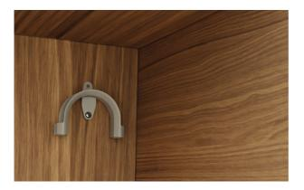
Install the drain hose support to the back wall, as close to the underside of the countertop as possible. Refer to 'Plumbing & electrical considerations' for minimum install heights.
