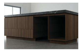
**4.** Ensure cabinetry floor is free from bumps and obstructions that could prevent the Dishwasher from sliding into the cavity.
